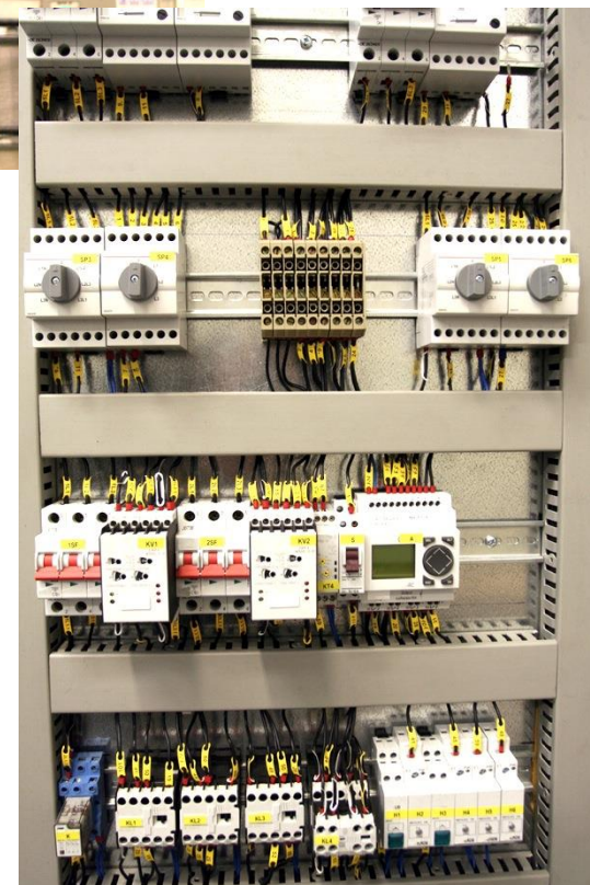
Control Panel field wired. Shutterstock
